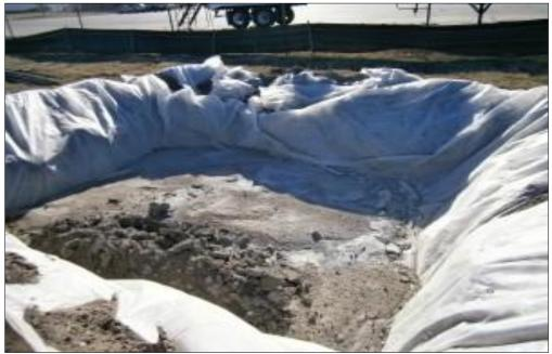
Plate 4-5 Concrete Wash Out Area
