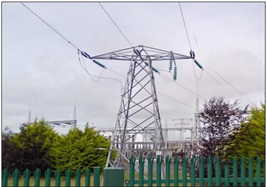
Plate 4-13 Completed End Mast Tower
