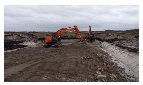
Plate 4-8 Internal roads under construction using the excavate and replace method. Source Bord na Móna.
