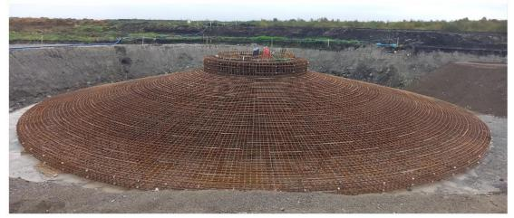
Plate 4-2 Turbine Base Anchor Cage
