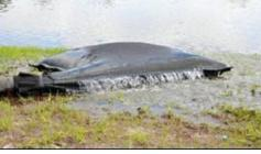
Plate 4-7 Silt bag under inspection
