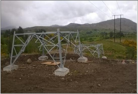
Plate 4-12 Steel lattice tower foundation complete
