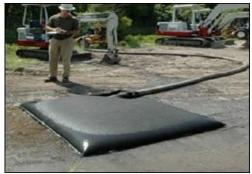
Plate 4-6 Silt Bag with water being pumped through
